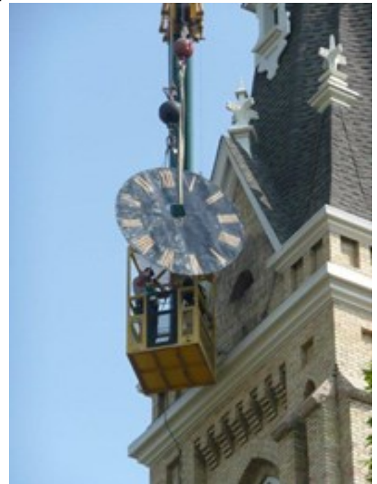
"Out with the old" Removal of one of the old clock faces.
