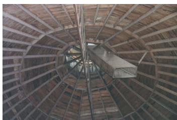
Ceiling of Lenneman Barn Aug 2001
